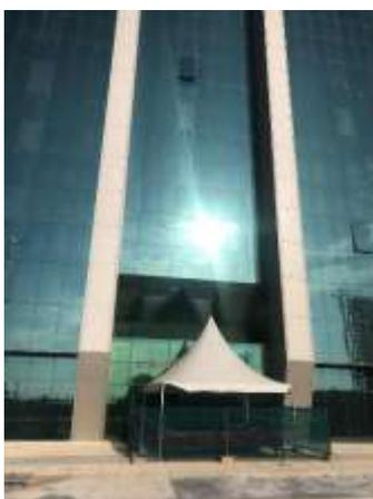
Olaya Tower 1 is an eight-storey with annex and two-level basement parking, mainly built of reinforced concrete structure. We were not able to inspect the offices areas due to on-going renovation at the time of inspection; however, external building finishes consist of glass curtain and aluminium cladding external façade, concrete exterior wall, glass on aluminium frame windows and main entrance door, marble elevator lobby wall, painted interior lobby wall and ceiling.
